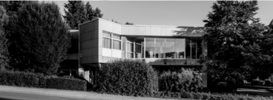
Avantgarde headquarter in Reichenbach, Germany
